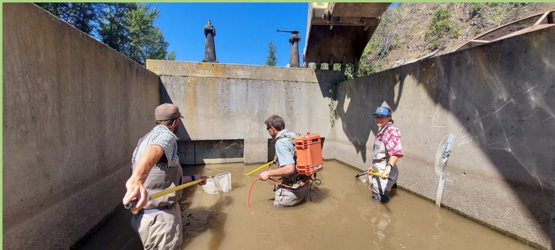
Katie helping relocate juvenile salmonids in July before a salmon habitat restoration project on a Methow River side channel that included removing the derelict concrete irrigation infrastructure seen in the photo.
