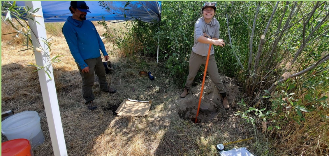
Working hard digging a ground water well.
