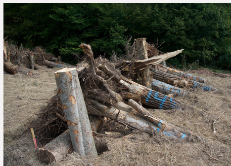
This roughened floodplain structure will slow down flood waters.
