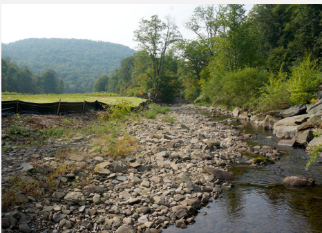
The berm at the edge of this field was removed, creating a more natural slope that will allow the creek to spread out over the floodplain during higher flows.
