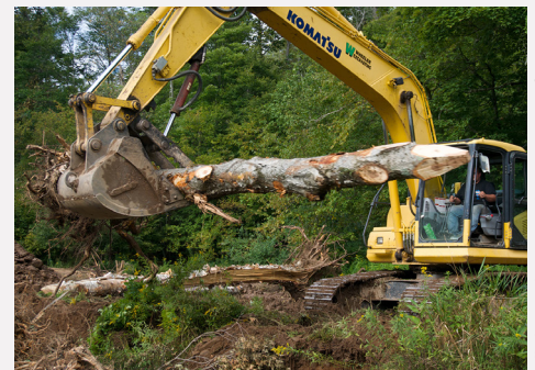
Crews placed logs and root wads at a number of locations to stabilize streambanks and provide fish habitat.
